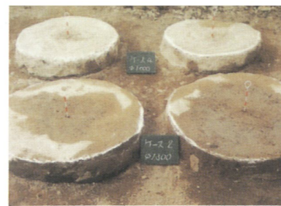
EX-DJM (拡大径翼杭施工)
