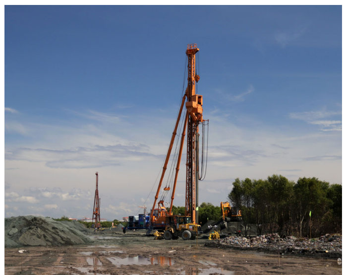
SCP project near Manila
