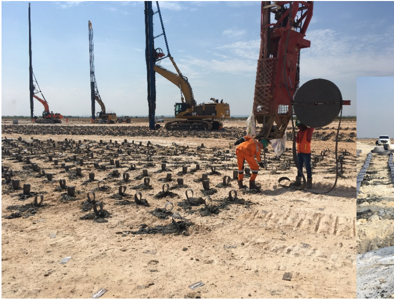
Wick drain rigs
