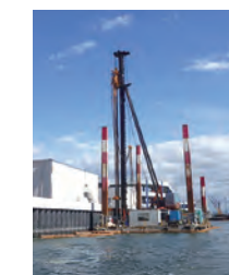
Barge-type rig: CI-CMC method
