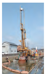
Barge-type rig: FTJ-NA method
