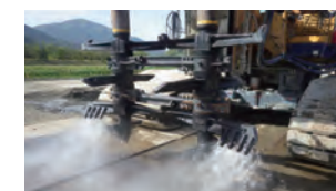
CI-CMC method: Ejector discharge and mixing blades
