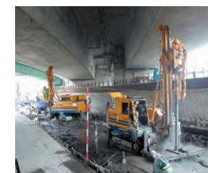
Ultra small rig: High-pressure jet mixing method
