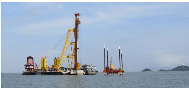
DCM barge and SEP for the core sampling in Hong Kong 2 nd Trial work
