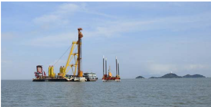
DCM barge and SEP for the core sampling in Hong Kong
